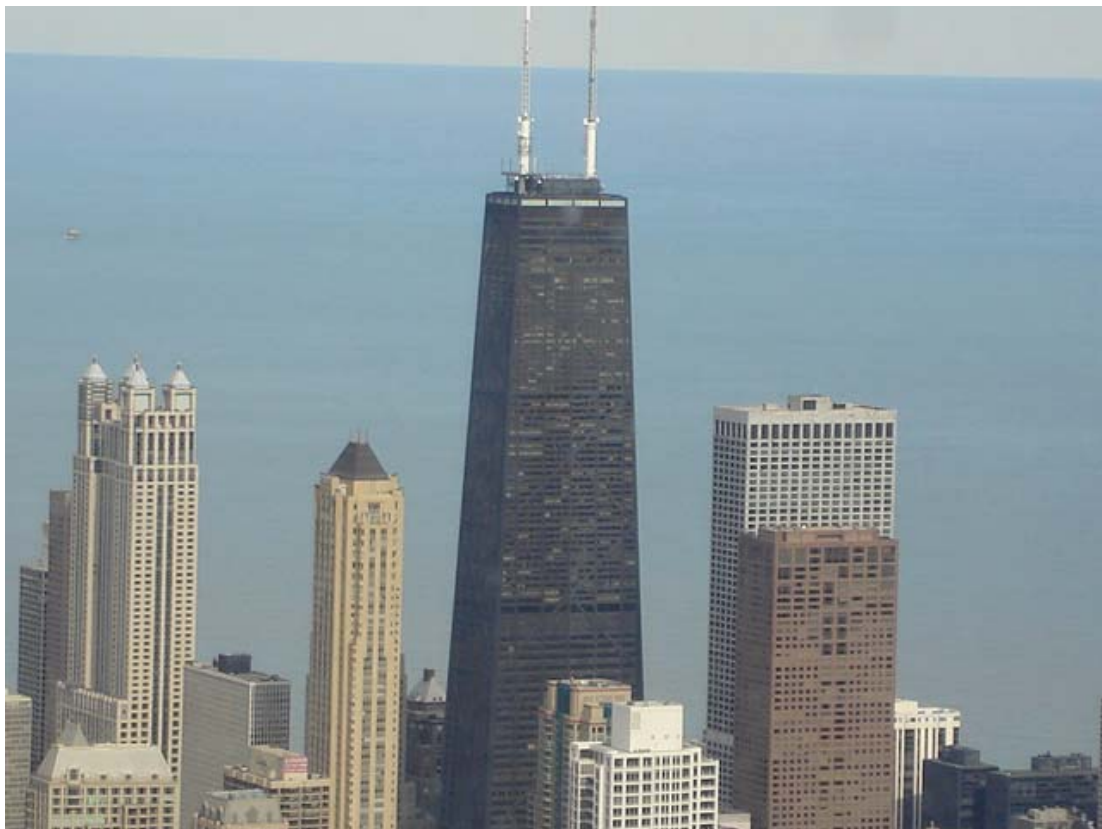
Fig 2: Close-up view of John Hancock Centre from Skydeck of Sears Tower (103 rd floor)
